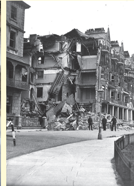
Granville Hotel showing bomb damage during World War Two. The west wing was destroyed and later rebuilt to more closely match the surviving end on the corner of Royal Road.
